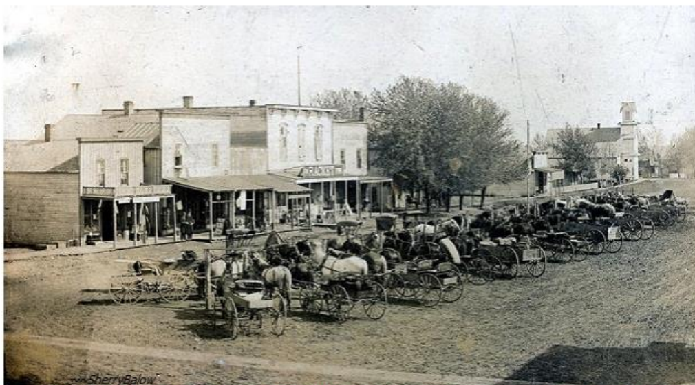
Weldon, 1890 - Joe Coffey Carpenter Shop, Charles DePew Section Foreman and Charles Pettis Blacksmith Shop "The Racket Market" 2nd from right of storefronts Photograph courtesy of Sherry Balow
